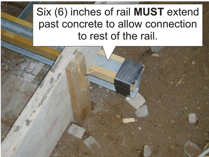
Six (6) inches of rail **MUST** extend past concrete to allow connection to rest of the rail.
