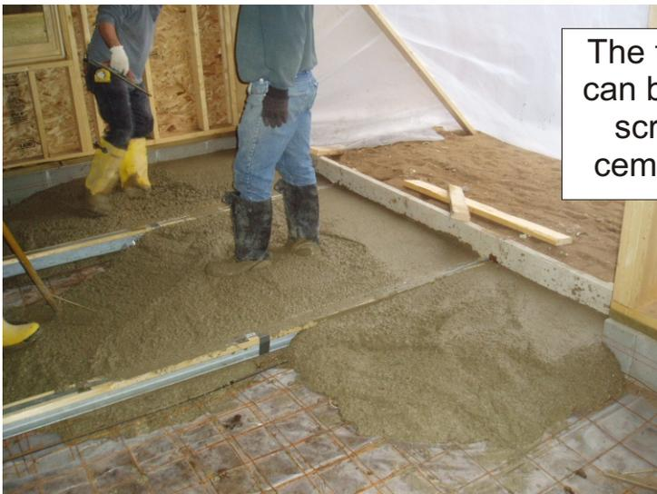
The track rails can be used to screed the cement level.
