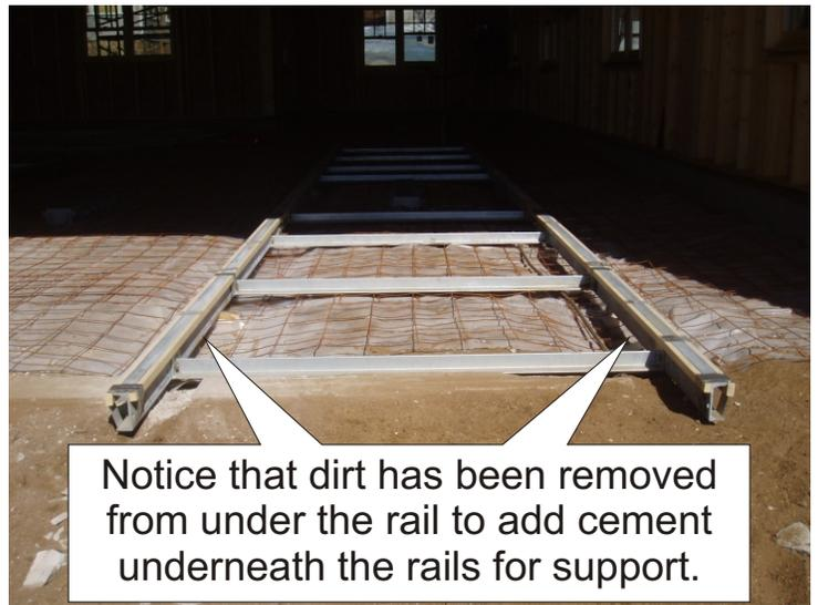
Notice that dirt has been removed from under the rail to add cement underneath the rails for support.
